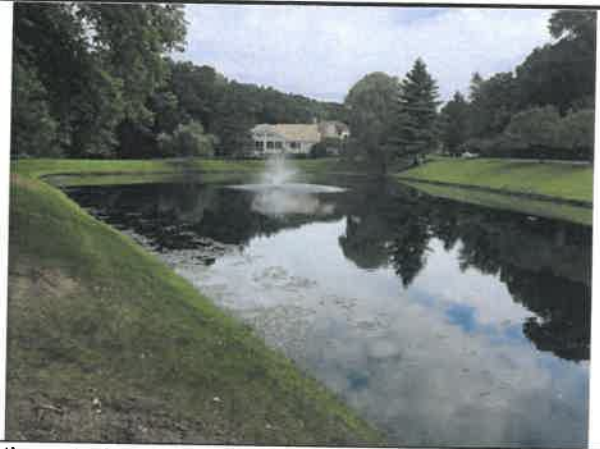
Southwesterly side of basin looking north easterly
