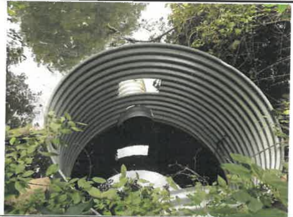
View into outfall structure
