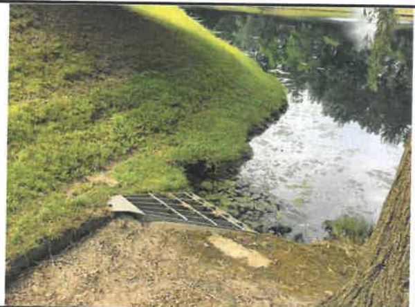
Area view of outfall structure
