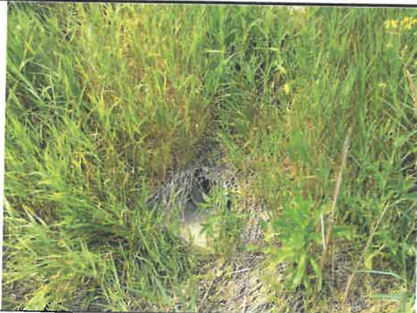
Side view of outfall structure
