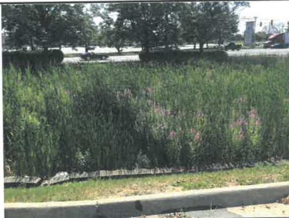
Westerly side of basin looking easterly
