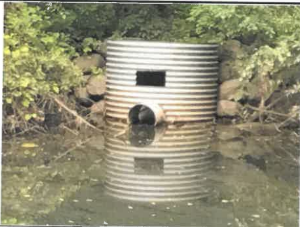
Easterly view of outfall structure looking westerly
