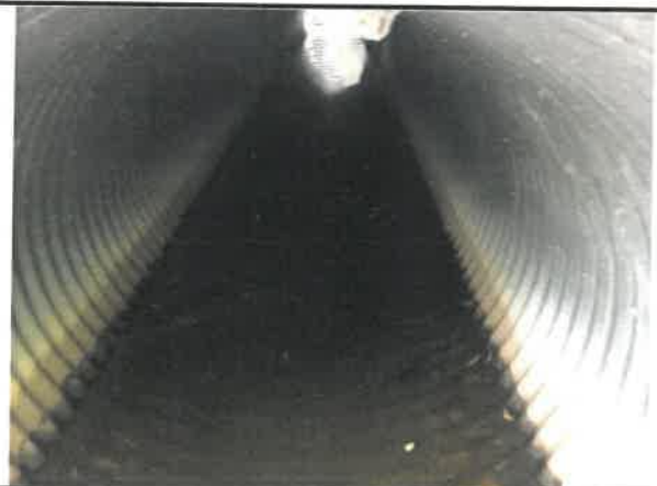
View into structure
