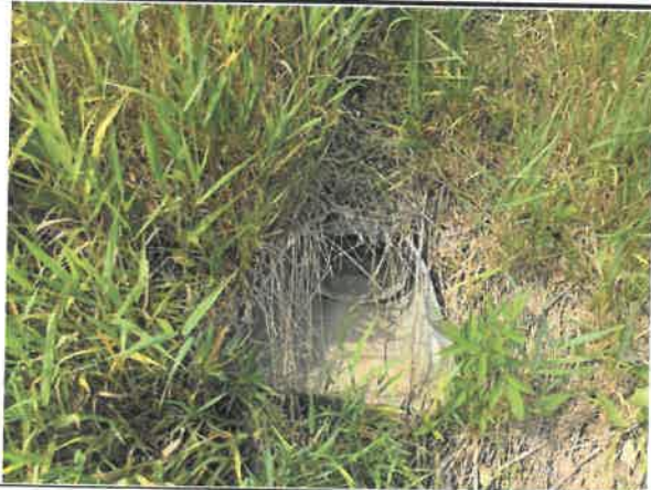
Front view of outfall structure
