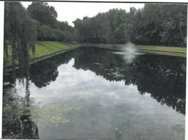
Northeastern side of basin looking south
