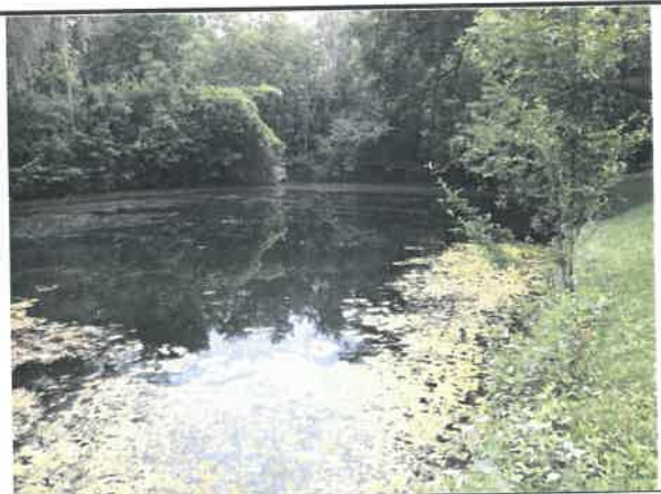
Southerly side of basin looking northerly
