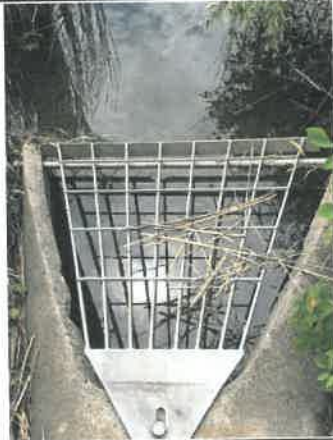
Top view of outfall structure
