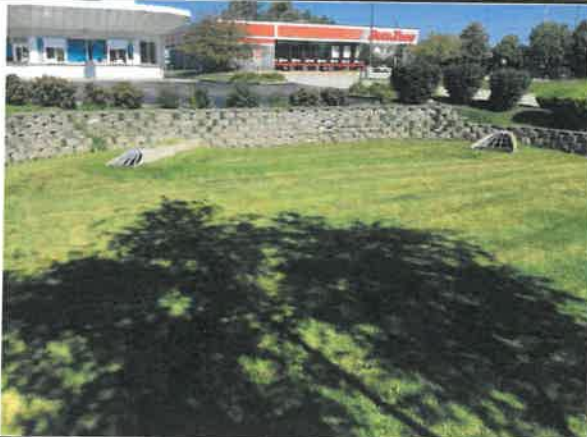
Southeasterly side of basin looking northwesterly
