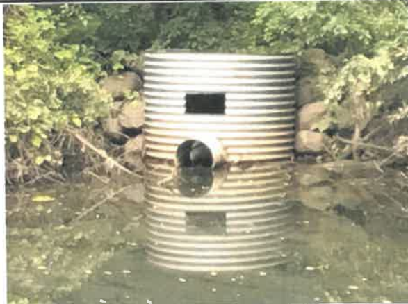
Easterly view of outfall structure looking westerly
