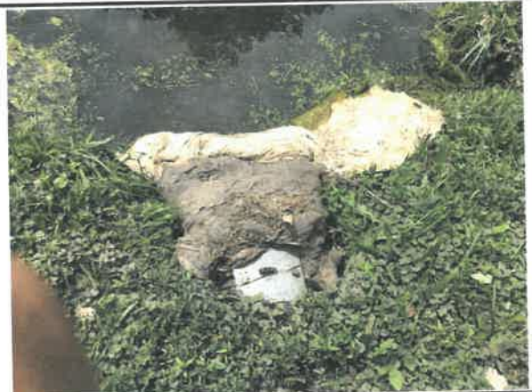
Completely sedimented due to wildlife
