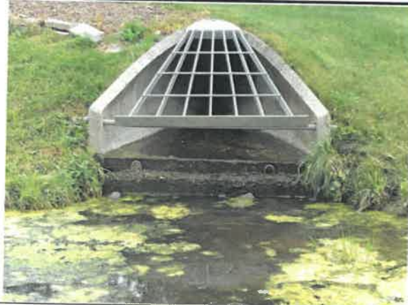
View looking into outfall structure
