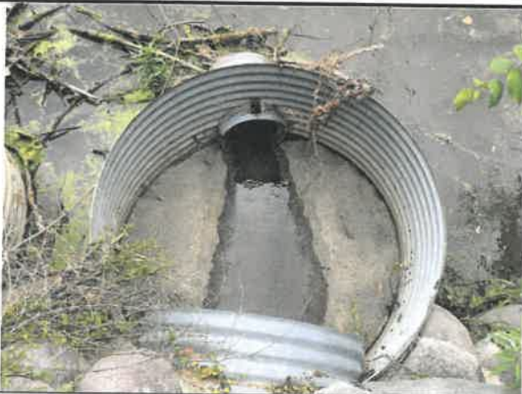
View looking down onto outfall
