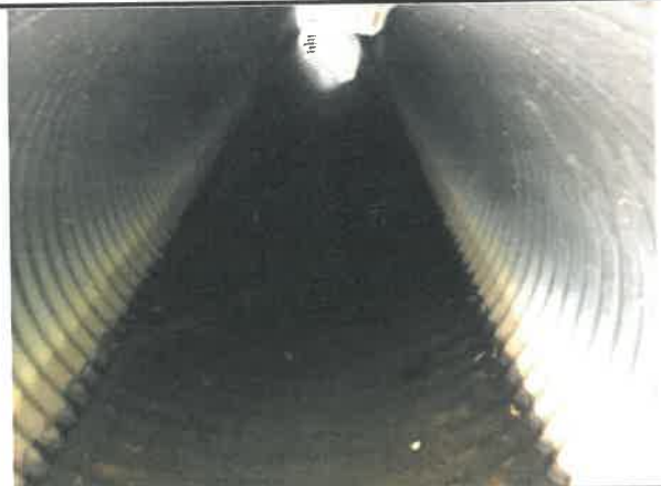
View into structure
