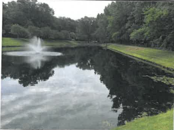
Northerly Side of basin looking south
