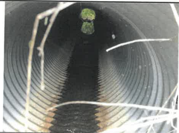
View into outfall
