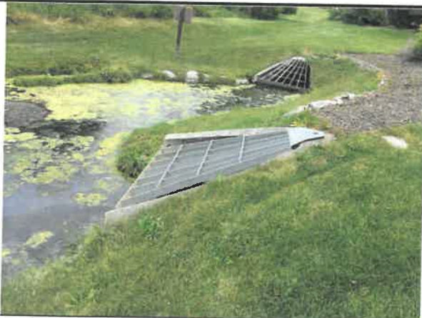
Side view of outfall structure
