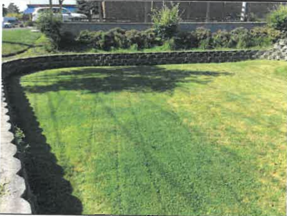
Northerly Side of basin looking south
