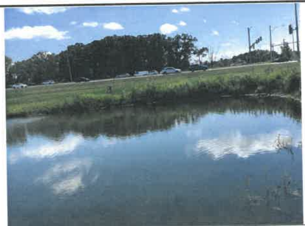
Northerly Side of basin looking south
