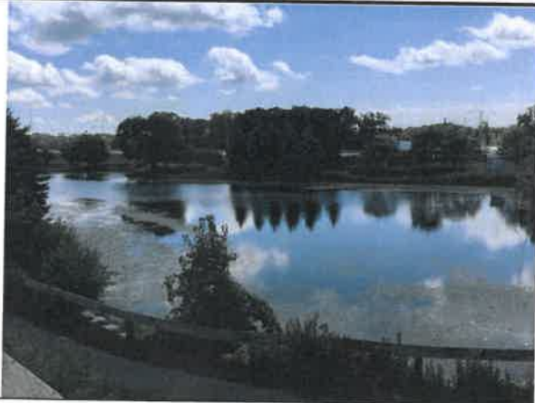
Northerly Side of basin looking south
