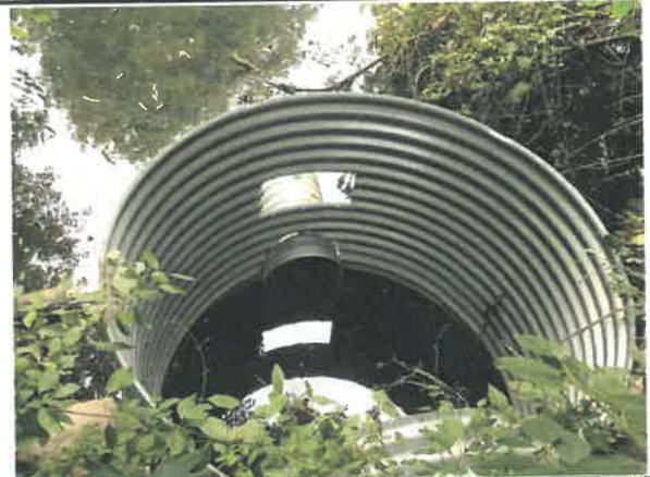
View into outfall structure
