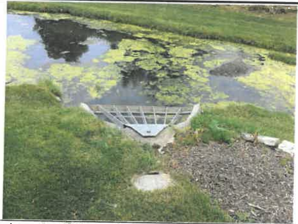
Top view of outfall structure
